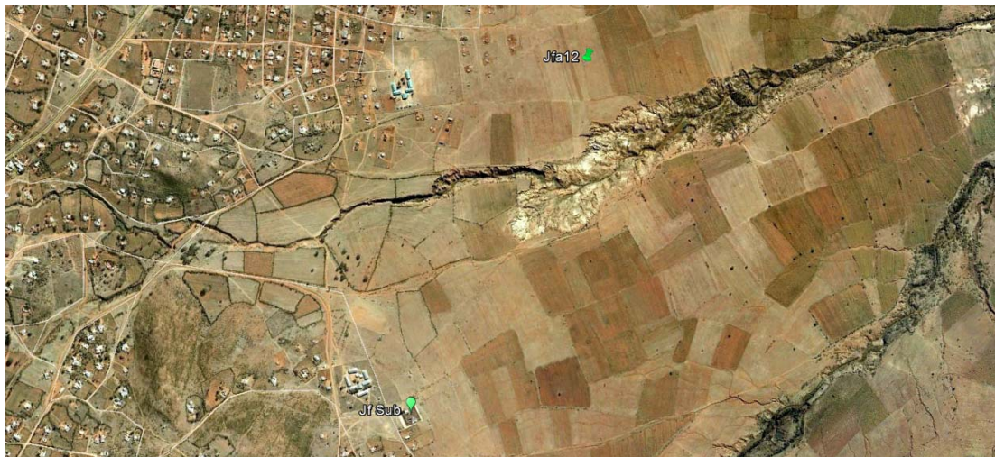
Figure 54: Close-up view of extensive erosion near the substation.
