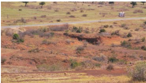
Figure 66: View along the corridor from the Tshatane substation sites – following the road south.
