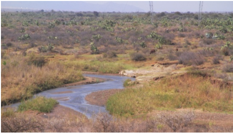
Figure 20: Crossing point of the power line over the Lepellane River to Jane Furse.
