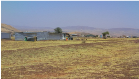
Figure 9: Example of erosion – increased runoff from hard surfaces.
