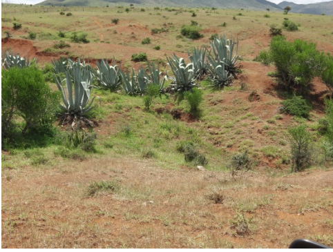
Figure 18: Drainage lines eroded – high flow velocity from hard surfaces in the residential areas.
