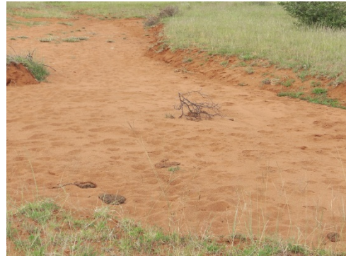
Figure 38: Example of erosion in vegetated area – run-off increase velocity.
