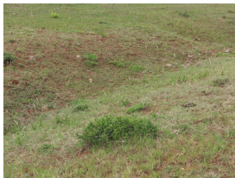
Figure 28: Some drainage lines with cover lowering erosion.
