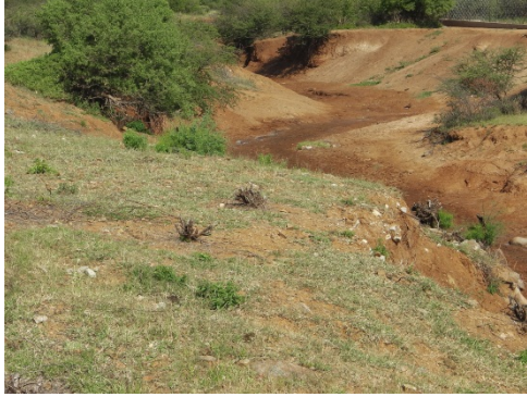
Figure 46: Increased erosion due to residential run-off – Apel.
