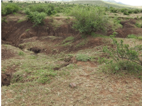
Figure 29: View of erosion on western bank of the Lepellane River.
