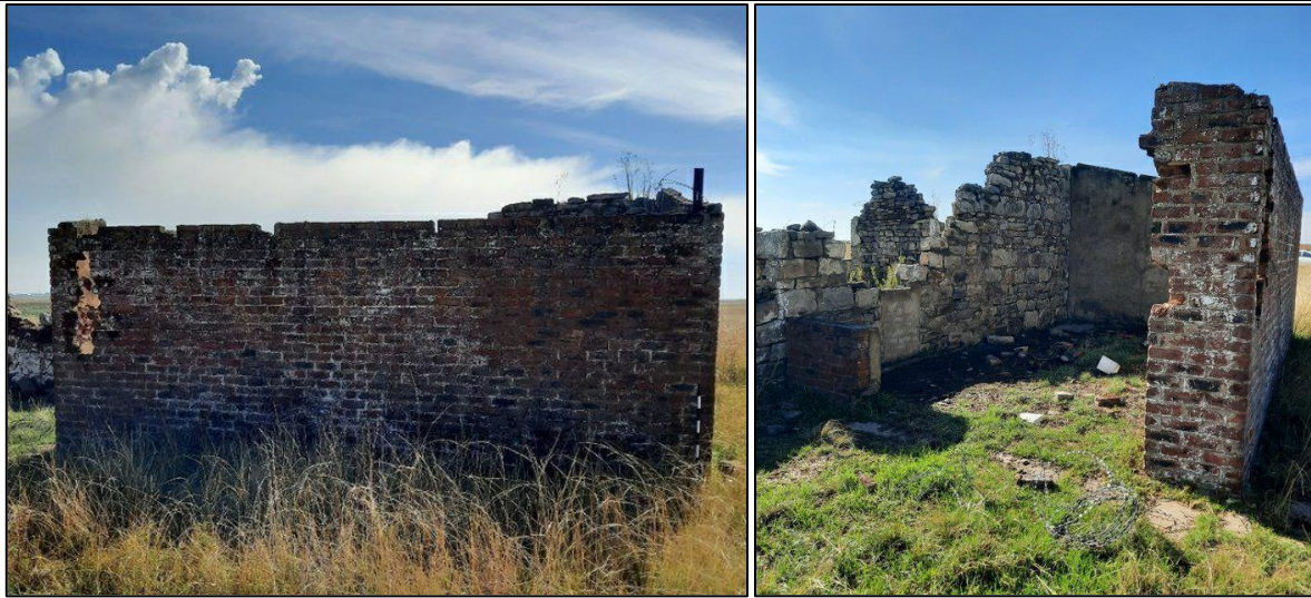
Figures 22 to 25: Four views of the main house showing the stone construction of the house and red brick walling of the added room.
