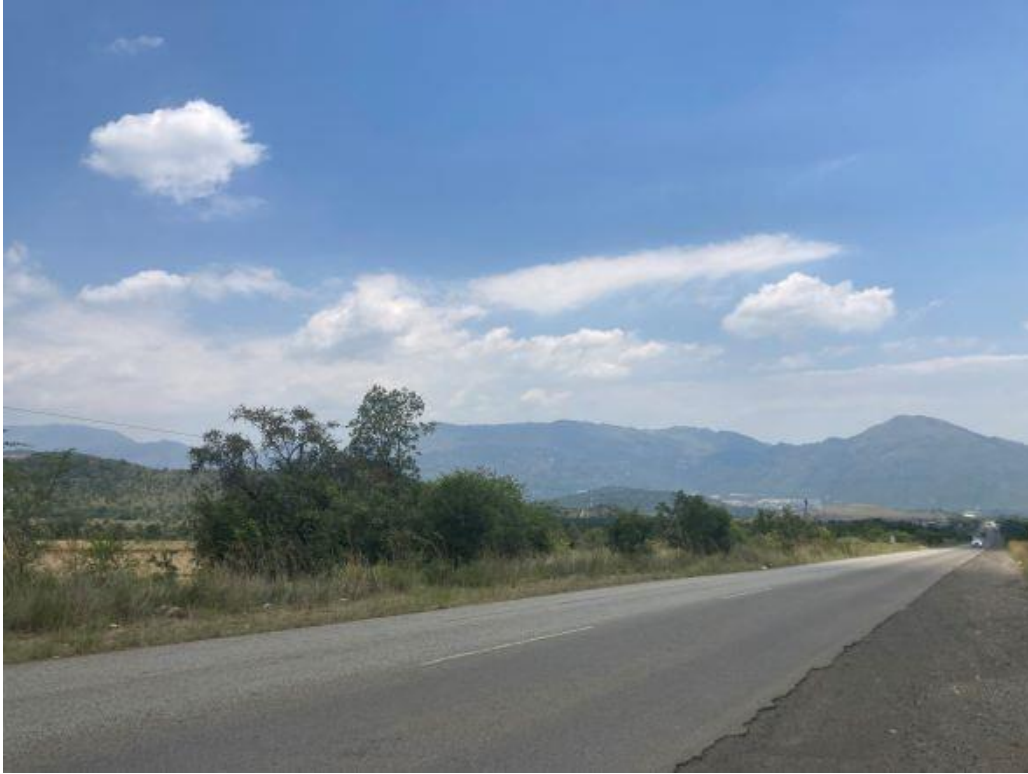
Figure 9: View of southern section of the proposed site
