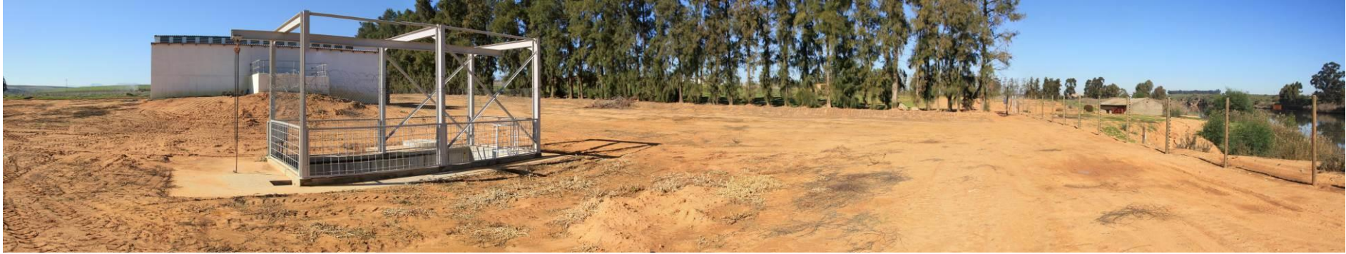
Figure 15: Example of pump sump situated away from the water resource (connected with pipes underground)
