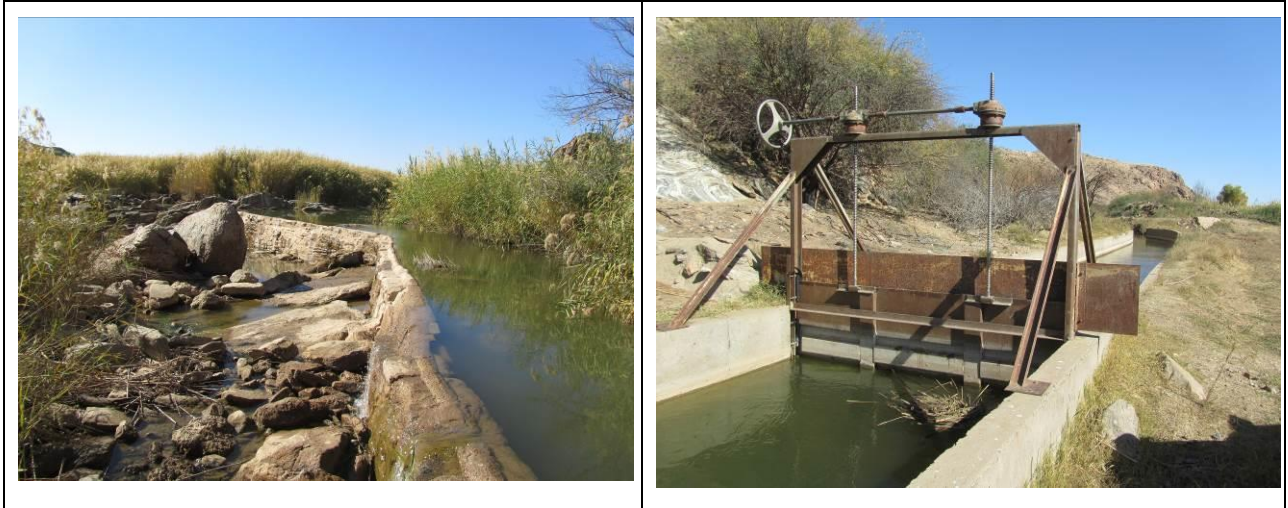
Figure 4c & d: Diversion weir and sluice gate at start of the canal
