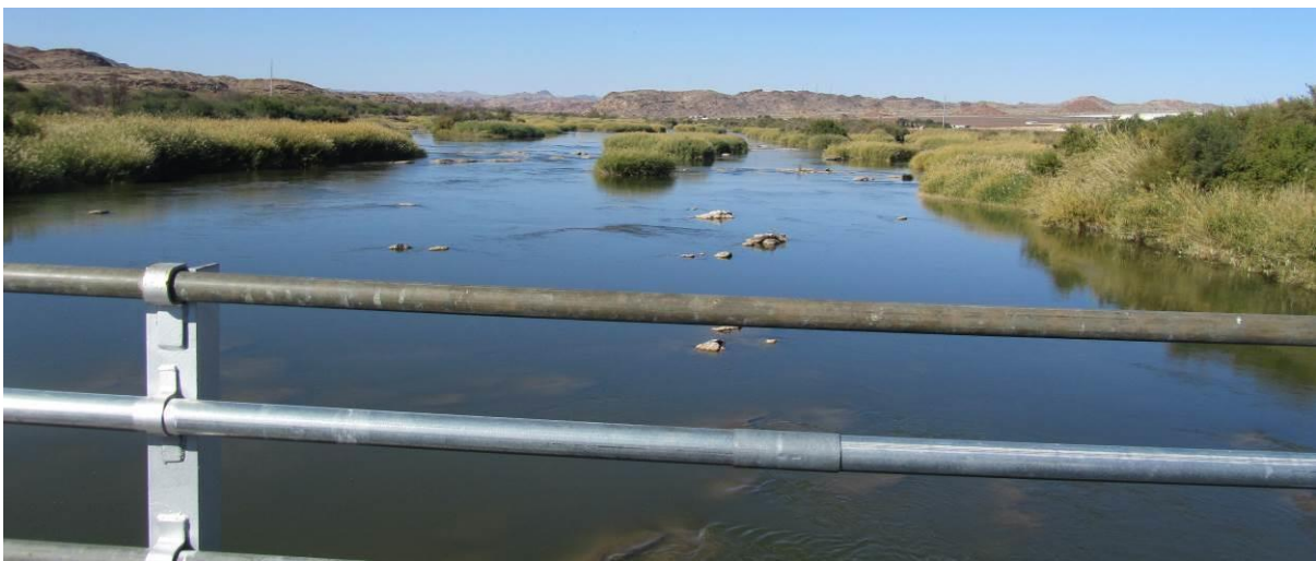
Figure 9b: Orange River at Onseepkans Border Post Bridge (upstream view)
