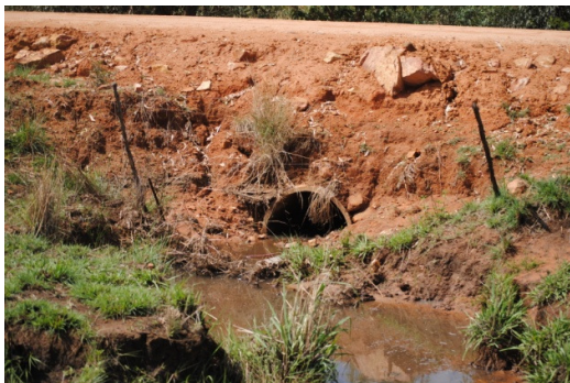
c) Stream flow under the gravel road.
