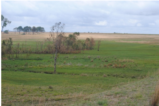
a) Seepage zone below reservoir wall.
