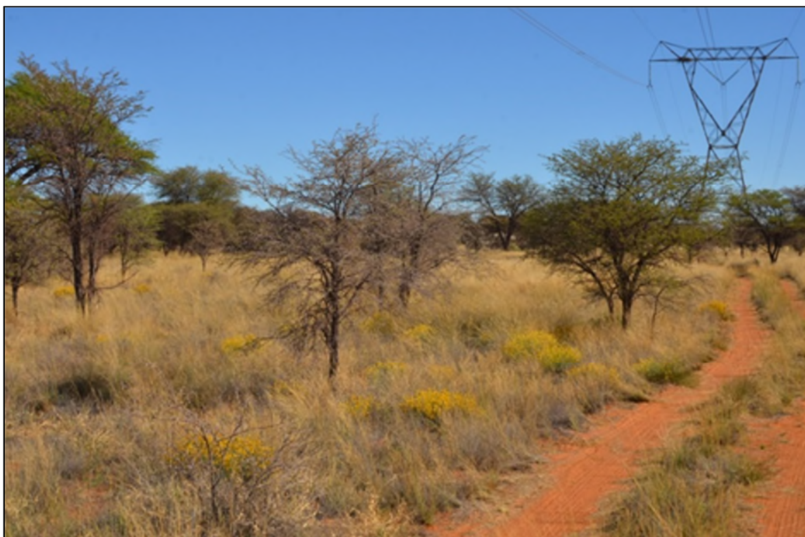
Figure 8. South of the Olifantsloop the density of Acacia erioloba trees remains relatively high, with an increase in younger trees. Note the large nest in the pylon, most likely constructed by White-backed Vultures ( Gyps africanus ), which are resident in the area.
