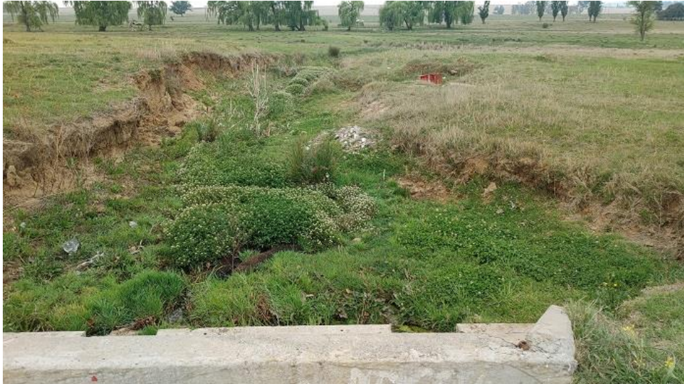
Figure 11: Image illustrating an example of the two small artificially/anthropogenically constructed stormwater flow channels, which will be traversed by the proposed pipeline route at the initial southern portion of the route
