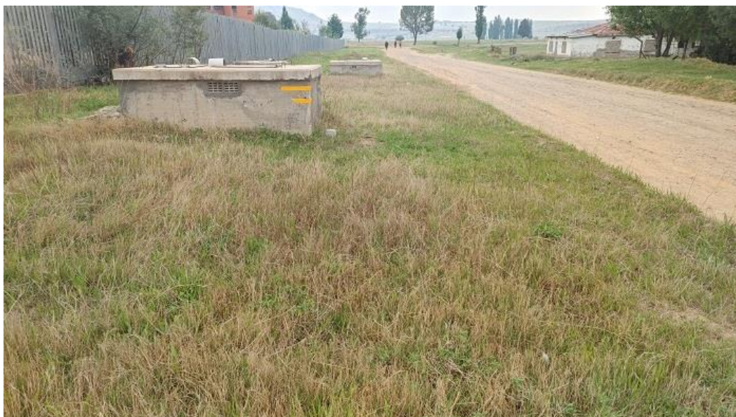
Figure 4: Image illustrating the moderate to highly disturbed and degraded anthropogenically managed state, associated with the short initial southern portion of the proposed pipeline route
