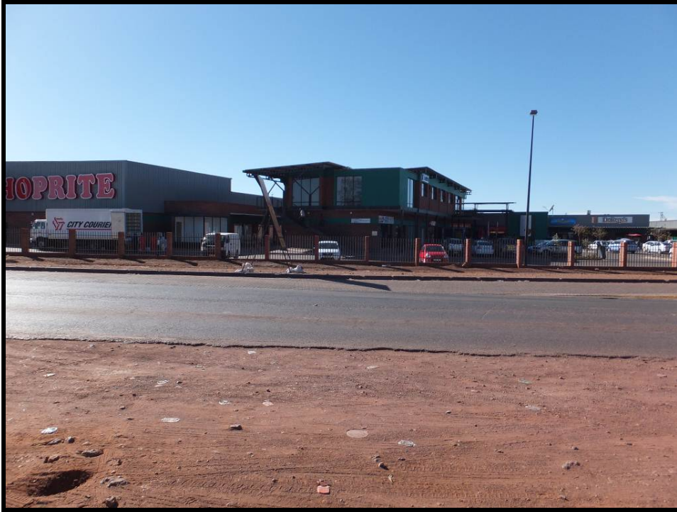
Photograph 2.6: View of Mall
