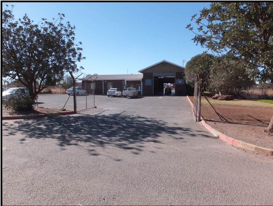
Photograph 2.5: Entrance to Traffic Department
