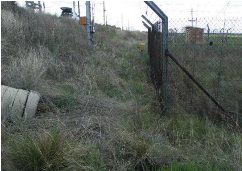
Photograph 4: Typical modified vegetation on the embankment and proposed substation locality
