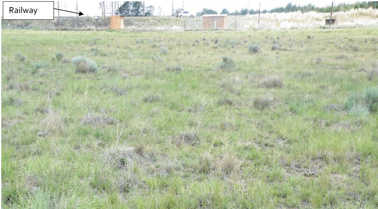
Photograph 2: View from the existing powerline southwards to the existing substation
