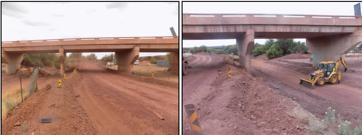
Figure 7: Representative photographs of Ga-Mogara River where the N14 crosses the river.
