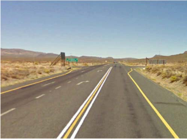
Photo 1: Eastbound view along the N1 towards the R354 intersection
