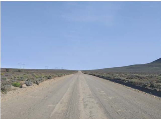
Photo 3: Westbound view along R355 towards the Loeriesfontein
