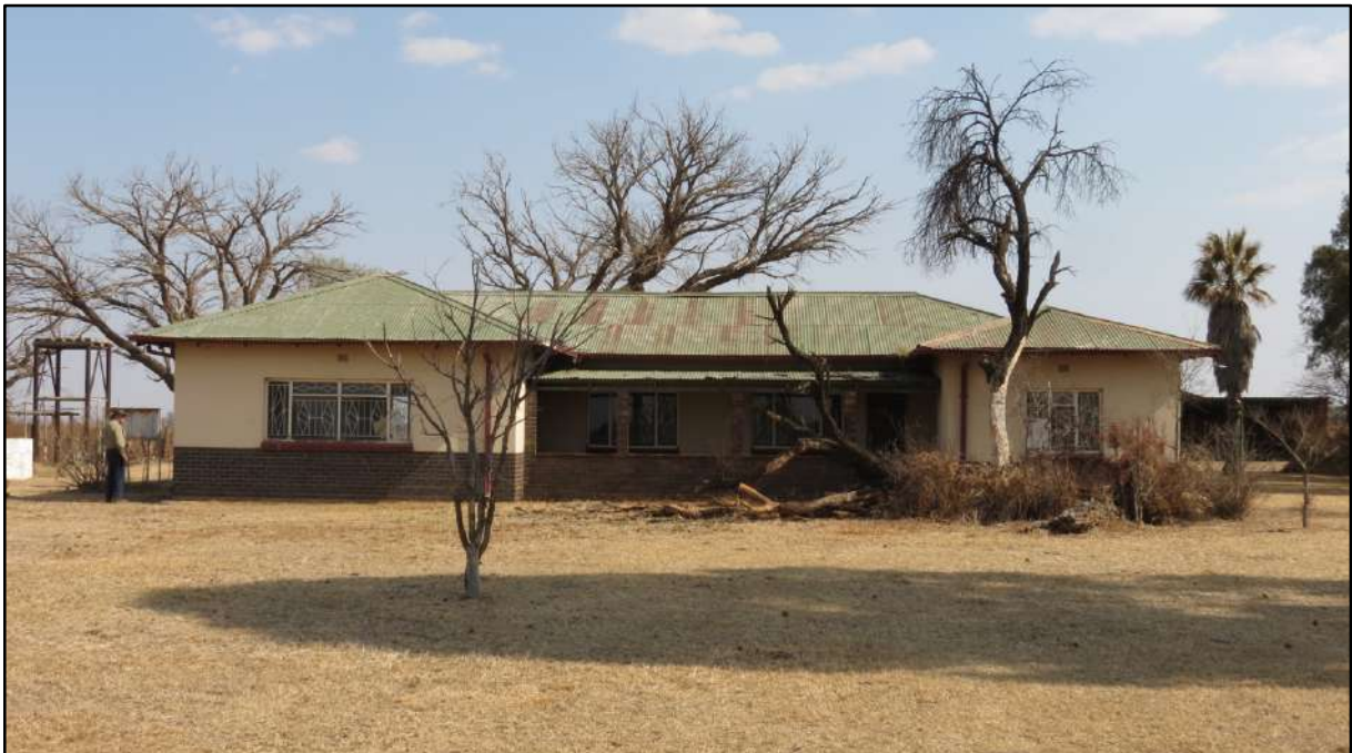
Figure 15 – This farmhouse was identified on the farm Kromdraai. An assessment of the available aerial photographs has revealed that it was built between 1961 and 1967, and as a result is not older than 60 years. This farmhouse is therefore not included in this report.
