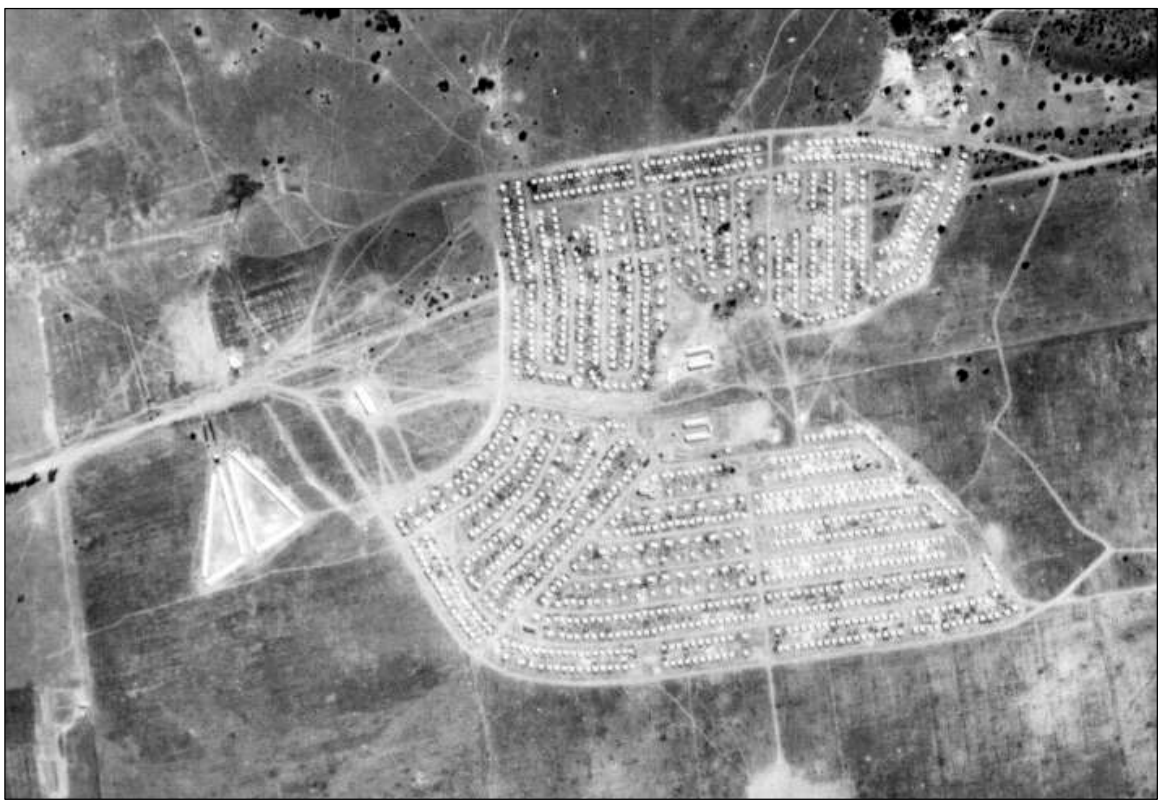
Figure 23 – This aerial photograph of Khuma Township was taken in 1961, roughly one year after it was established (NGI, Aerial Photographs, 425_021_02738).
