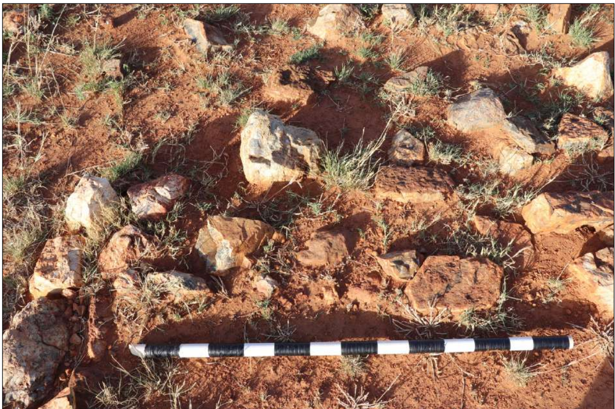
Figure 60 – Closer view of a section of walling from the structure. Scale in 10cm increments.
