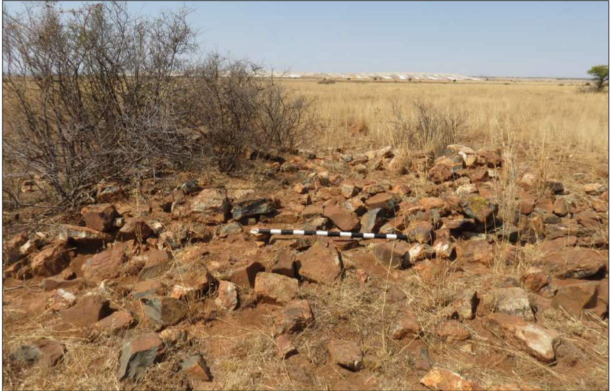
Figure 42 – General view of the structure at site AGA-MWS-WBP-3A. The existing Kareerand TSF can be seen in the back. Scale in 10cm increments.
