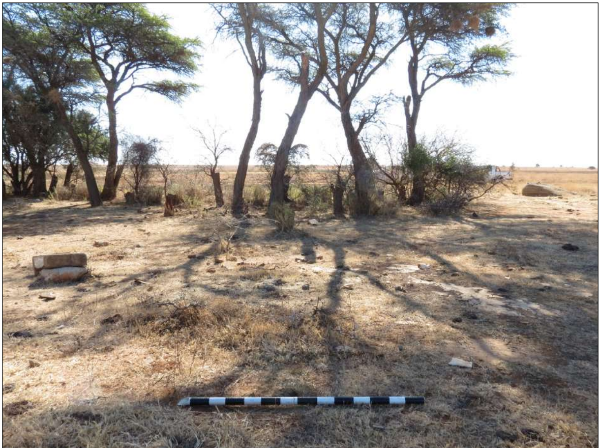
Figure 35 – General view of the rectangular cement structure at site AGA-MWS-WBP-1. In the background, a section of the clump of camelthorn trees can be seen. Scale is in 10cm increments.
