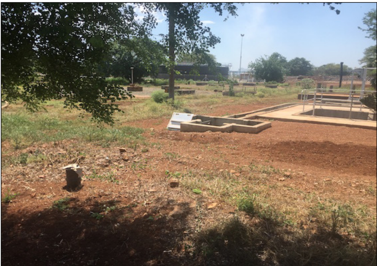
Figure 4: Existing infrastructure on site.
