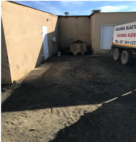
Photo 5: BH_CA2, Buried underground
