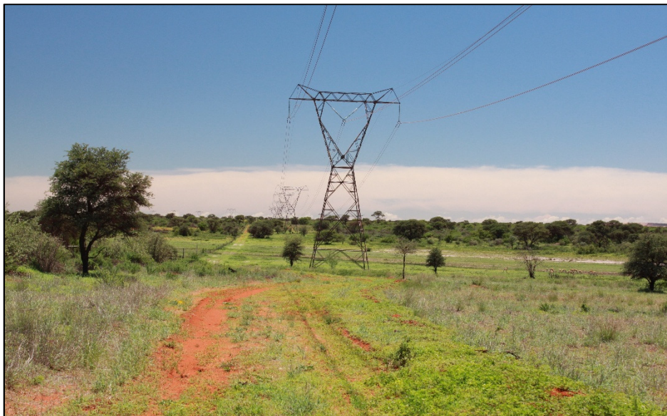
Figure 10: The 275kV power line as well as service road crossing the Ga-magara river.
