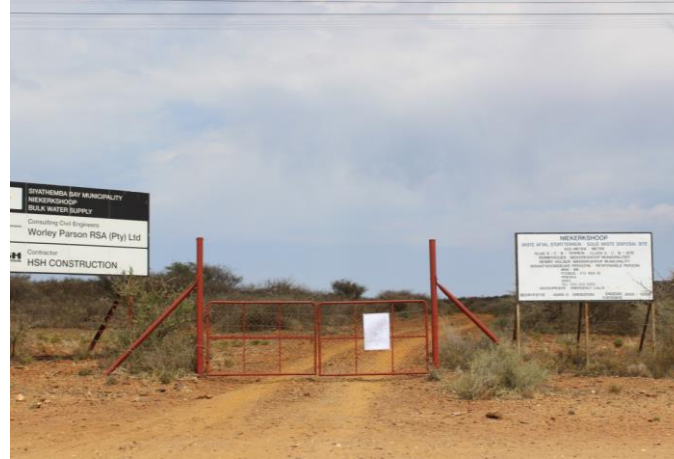
Figure 2: Site Notice at the main entrance gate (along the R386) leading to Niekerkshoop landfill site
