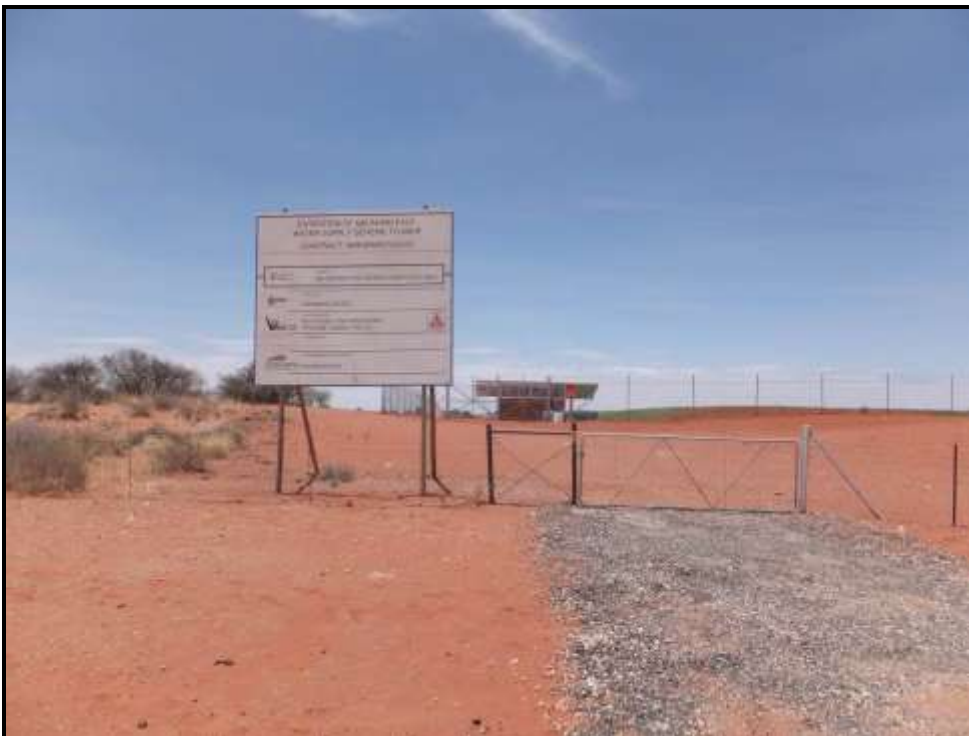
Photograph 1.7: Kalahari East Water Pipeline
