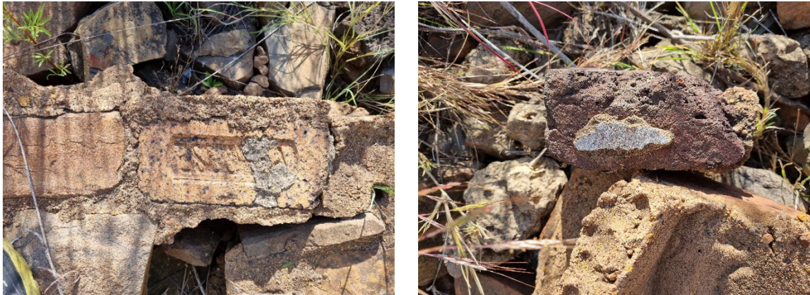
Figure 24: stone structures indicating the use of local stone, brick, cement and metal.
