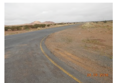
Picture 3 – Looking right from MN73 (the existing and proposed construction access)
