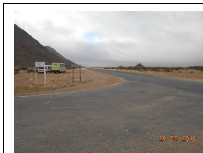
Picture 1 – Looking left from MN73 (the existing and proposed construction access)
