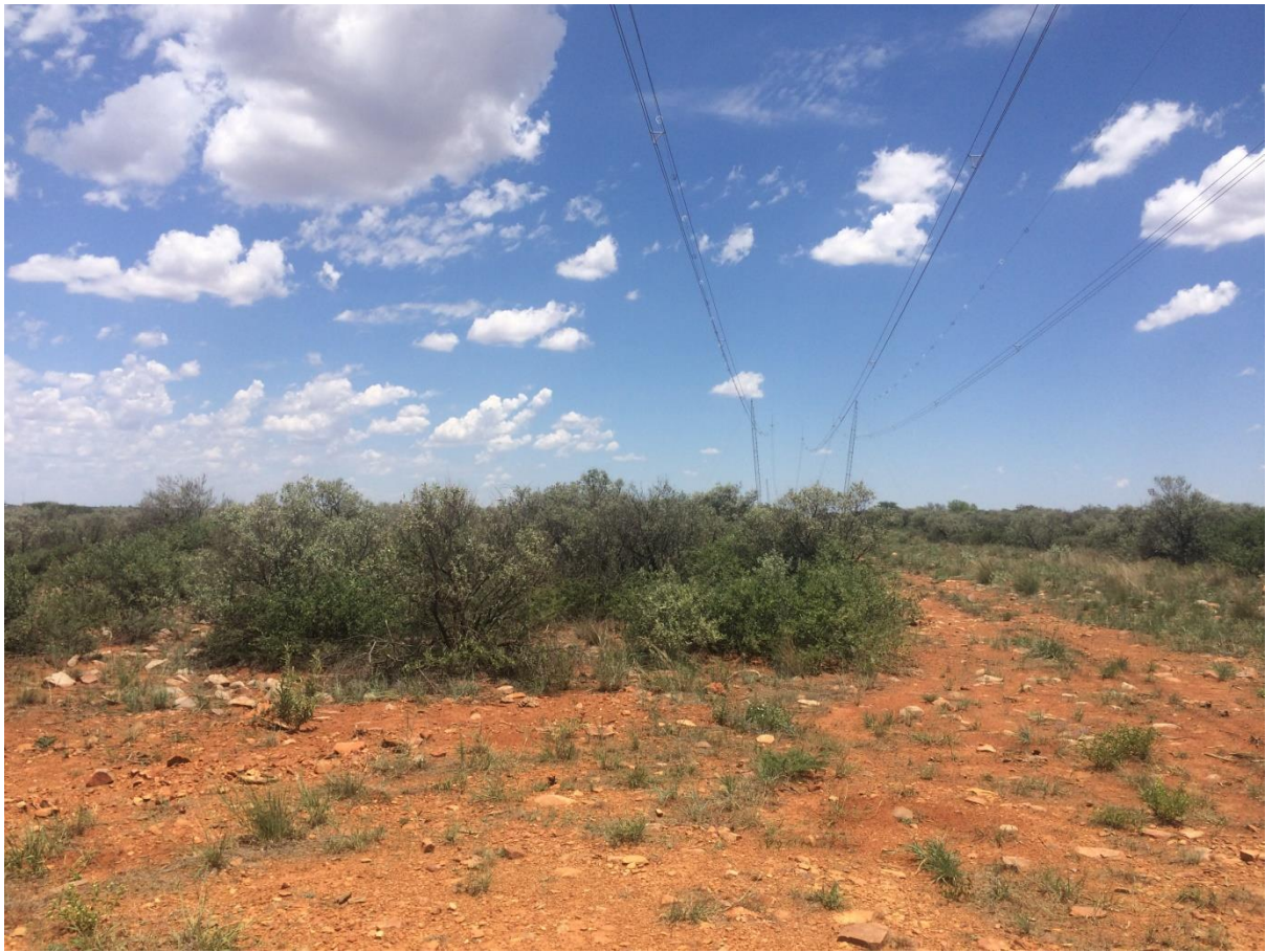
Figure 7: View of Mookodi Mercury 400kV power line
