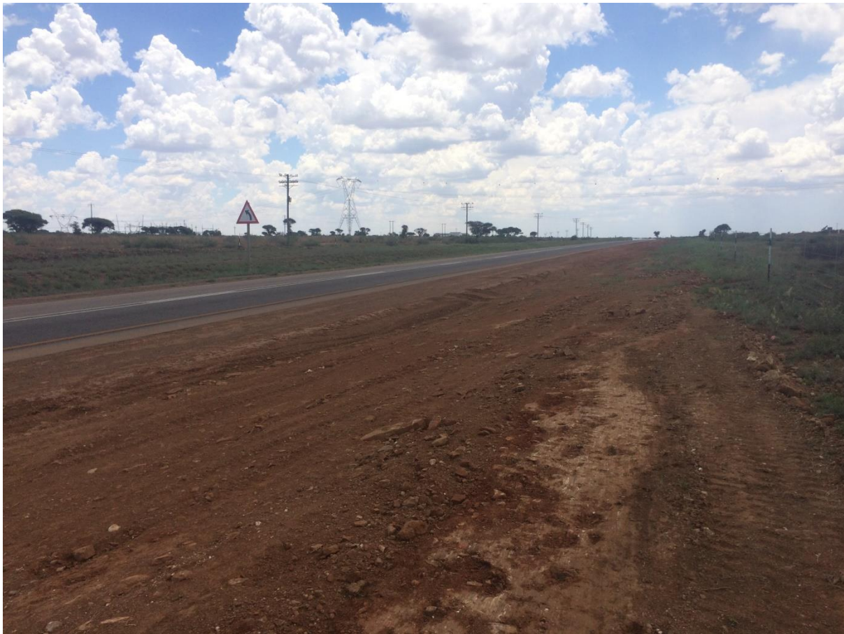
Figure 8: View of N18 national road crossing and towards Vryburg
