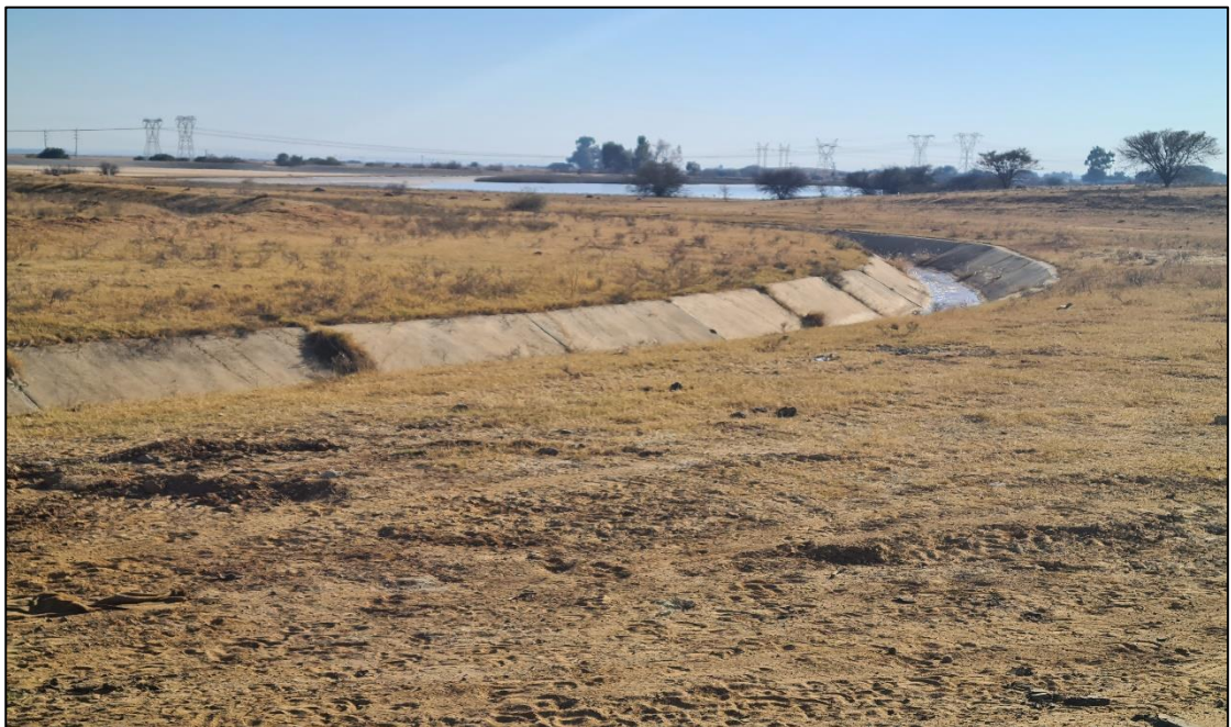
Photograph 3. Man-made dam and concrete canal in the project area
