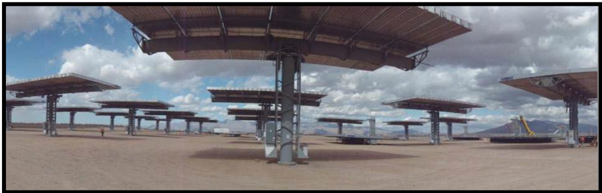
Photo 8: Typical layout of such a solar site (Image courtesy of Amonix, a leading designer of CPV technology)
