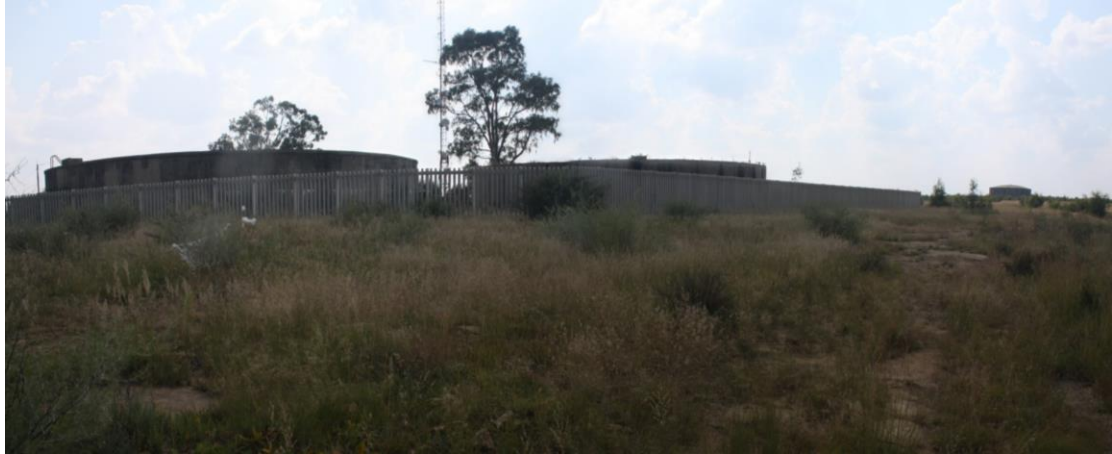
Figure 5: View of the water reservoirs on top of the sandstone hill where the pipeline will connect to.
