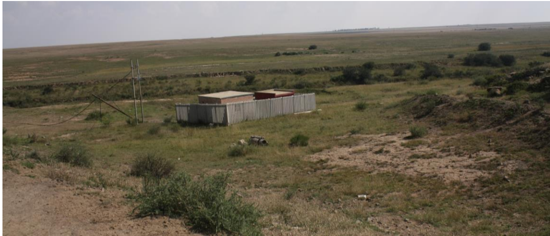
Figure 8: View of the pump station at the Senekal Dam where the pipeline will connect to the system.
