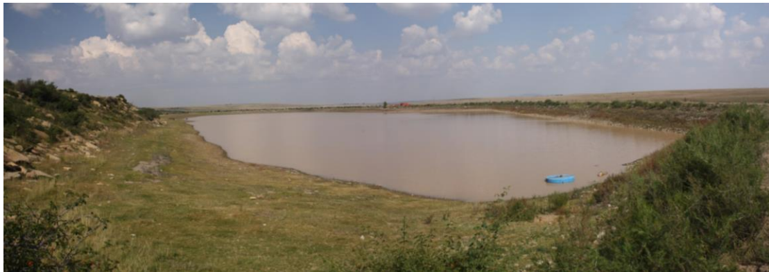
Figure 9: Panorama of the Senekal Dam at the southern end of the pipeline route.
