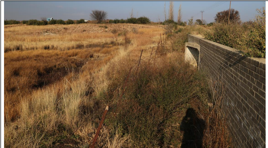
View of the culvert over the stream at the point of crossing. This also contributes to modification of the flow and flooding regime and ponding upstream of the culvert.
