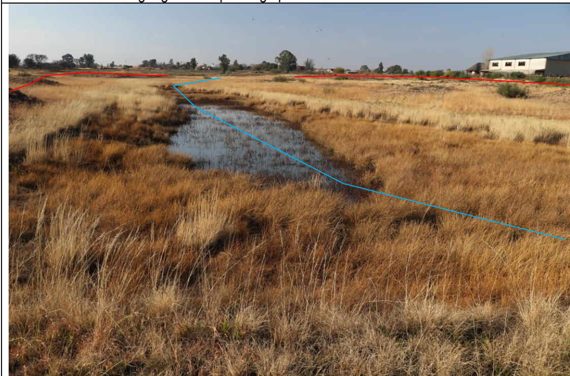
View of the stream upstream of the point of crossing. Note clear ponding caused by the road crossing. The flood bench is also quite visible here (red).
