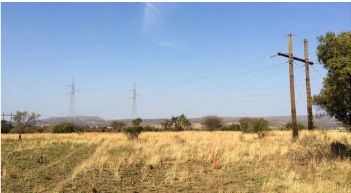
Figure 17: Photograph 4 in a northerly direction of the Alternative 2 substation location and the southern section of the Alternative 2 power line routing.
