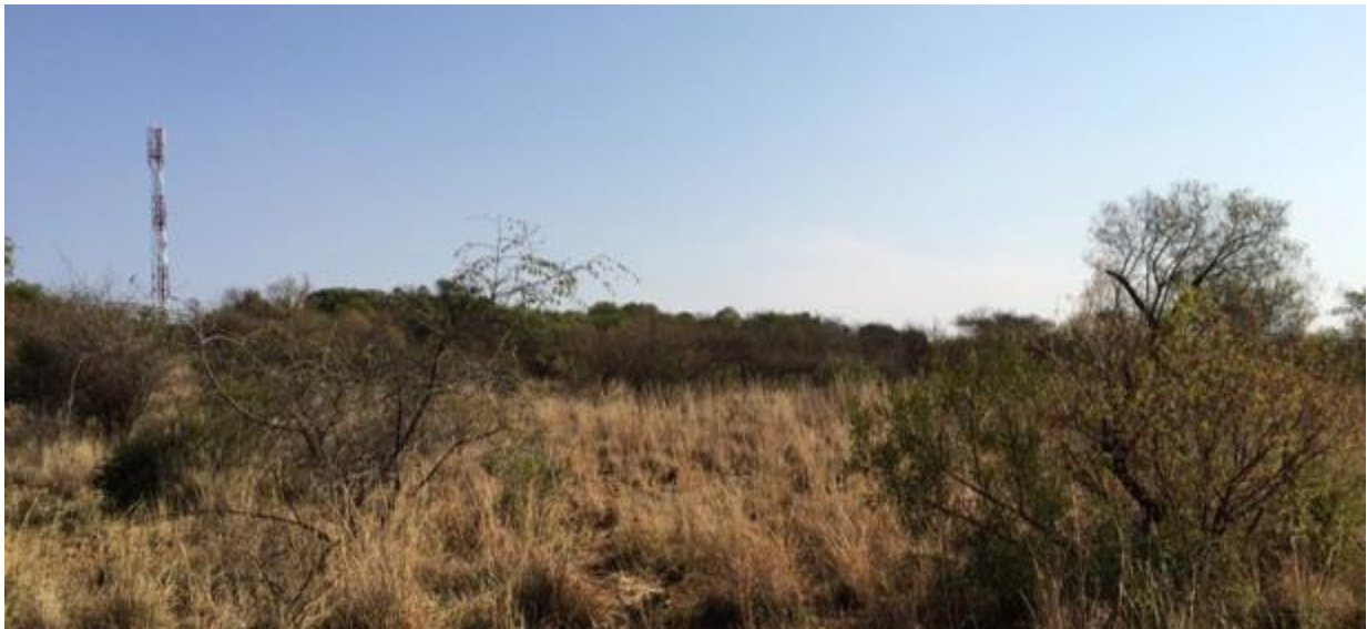
Figure 14: Photograph 1 in a southerly direction depicting the Alternative 1 substation location with the cell tower in the background.
