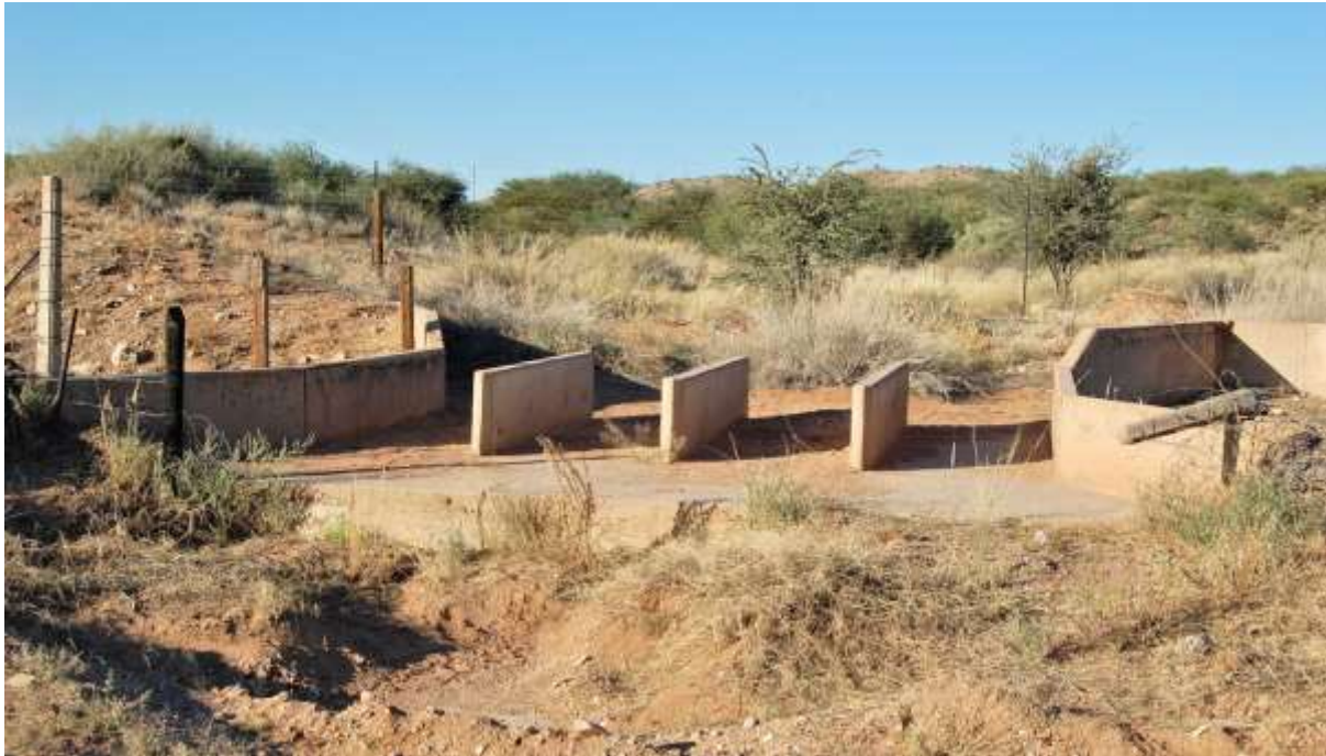
Figure 14 Drainage line crossing irrigation canal
