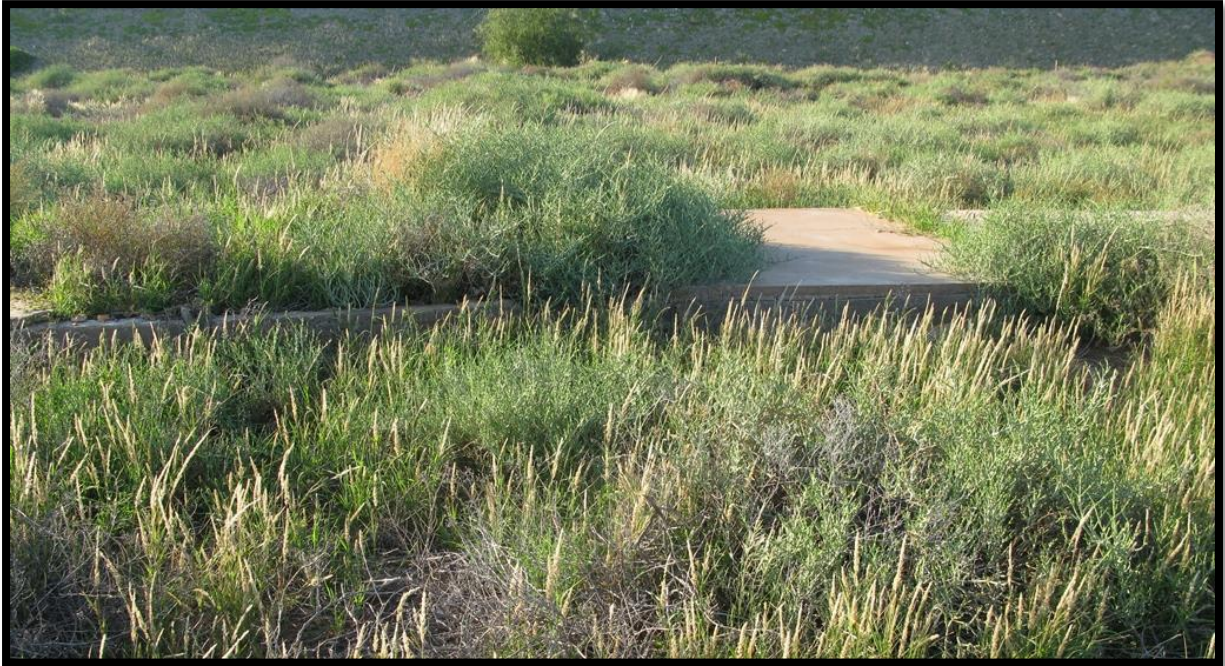
Photo 3: Photo showing one of the old foundations found within the Mesembryanthemum veld
