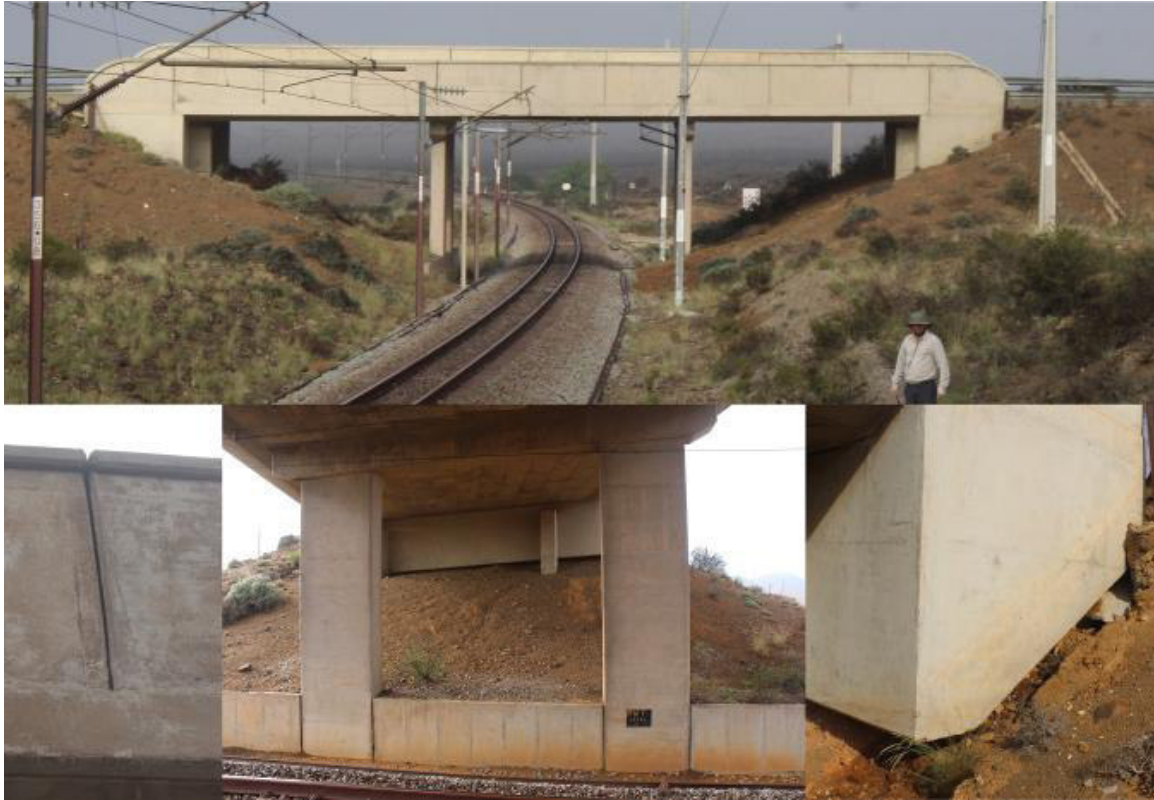
Figure 3-21: Photographs of the railway road overpasses and features relevant for potential bat roosts.
