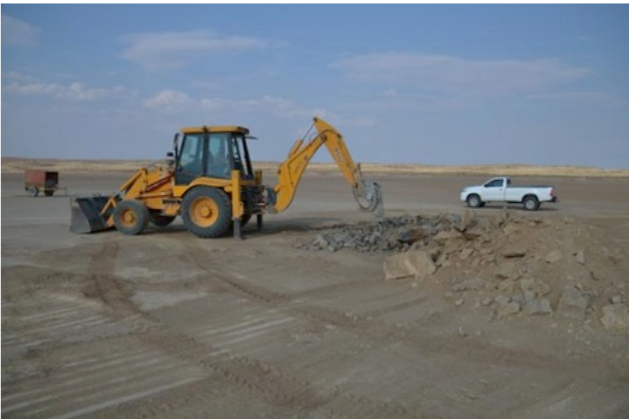
Figure 39 Excavation process on Hakskeenpan
