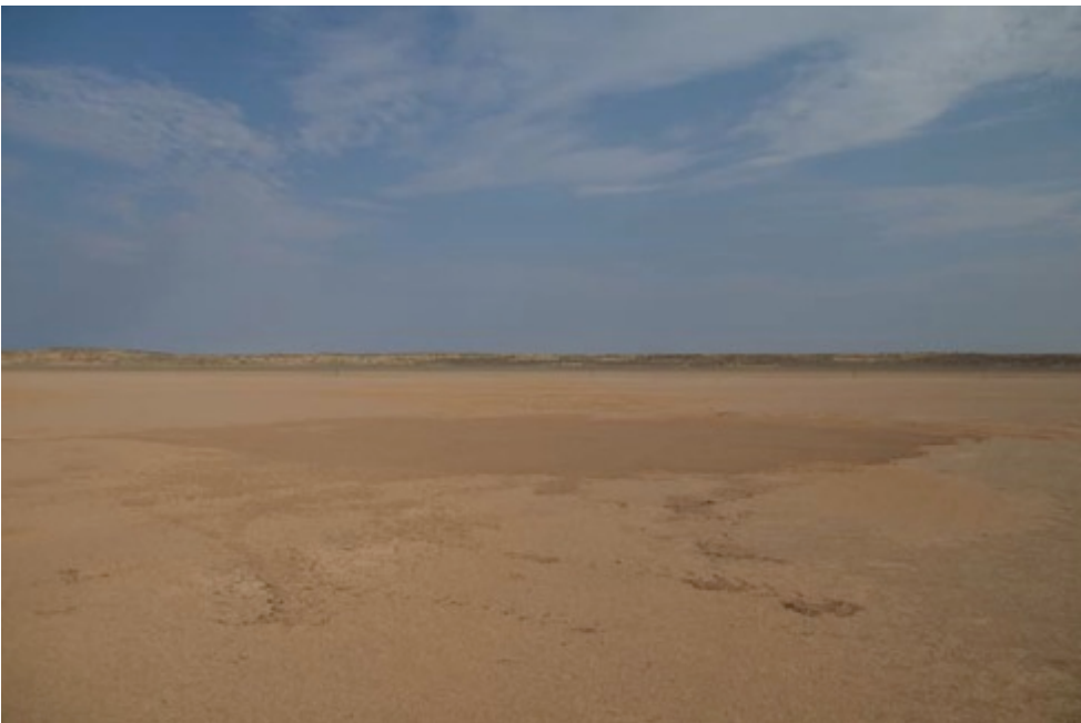
Figure 41 Completed in-filling and graded section on Hakskeenpan
