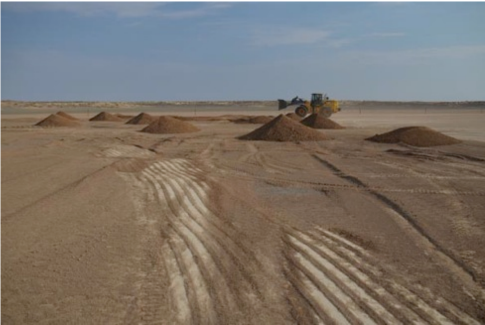
Figure 40 In-filling and levelling process on Hakskeenpan
