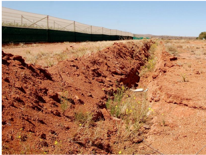
Figure 7 Cut-off Trench
