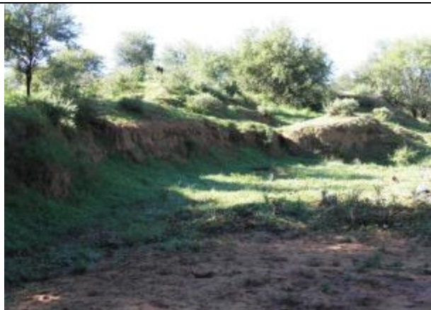
Photo 1: The deep eroded channels of the upper portion of the Olifantsloop watercourse.
