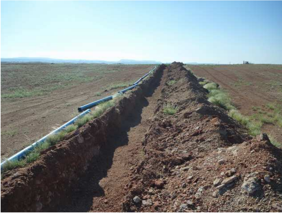
Figure 15 Trenches for the laying of irrigation infrastructure
