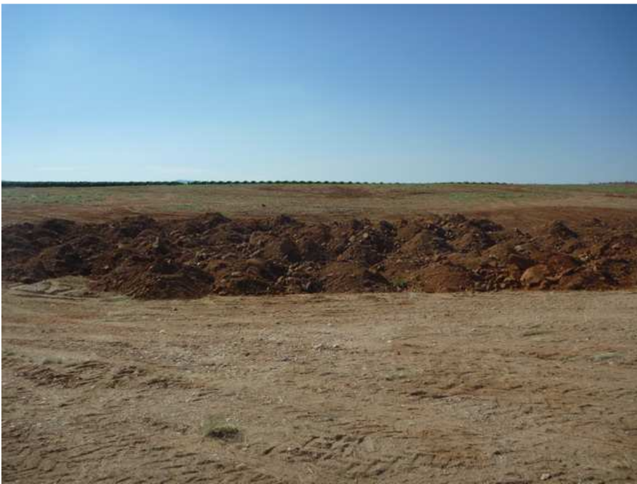
Figure 10 Dumped soil material for levelling purposes
