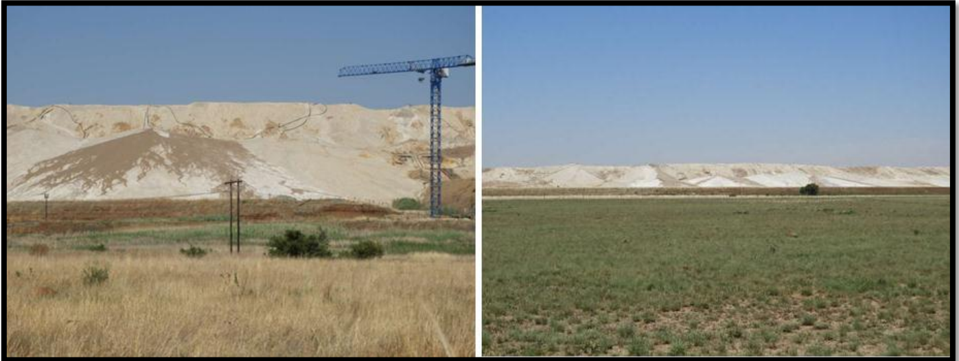
Figure 25: The operational tailings storage facility.
