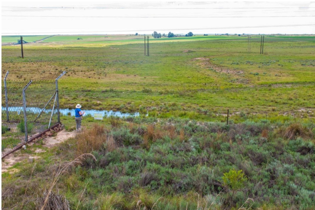
Figure 4: A north-westerly view from the railway line, overlooking the grassland towards the existing powerline to which the new substation will be connected. The figure in the image provides scale to judge the length of the in/out lines. Note the manmade furrow that holds water seasonally.
