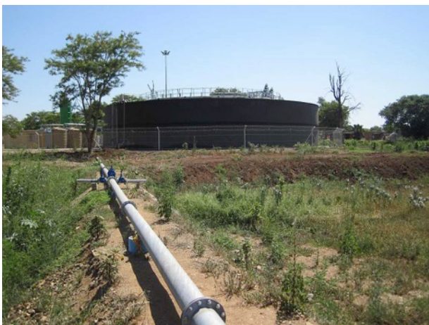
Figure 6 – View of infrastructure on site
