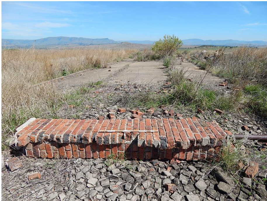
Fig. 44: Recent infrastructure which has been demolished. Only a concrete slab and rubble are left (R 1). This structure was situated next to the air strip.
