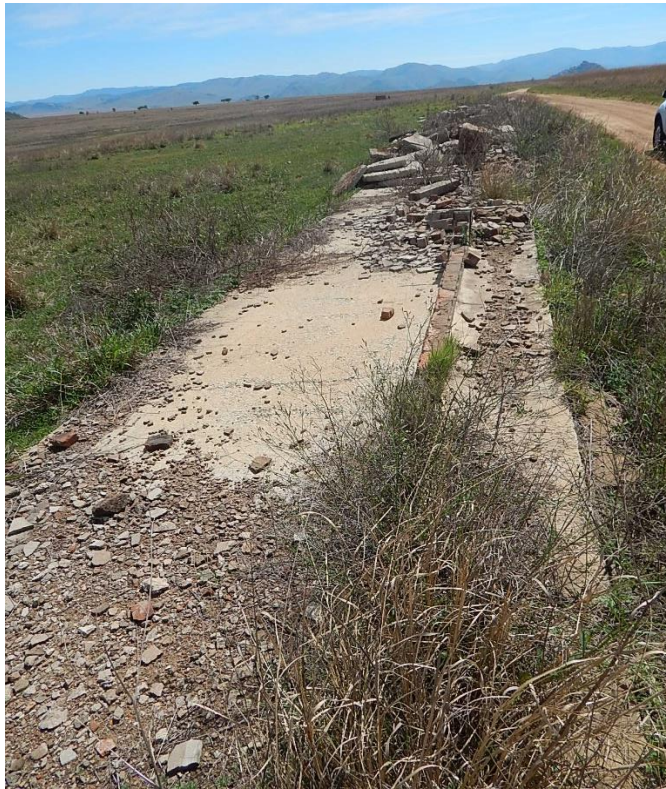
Fig. 46: A recently demolished structure. Only a concrete slab and rubble is left (R 3).
