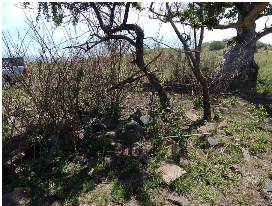
Fig. 54: The indistinct remains of a LIA stone wall (LIA 7), next to an access road. This structure has been severely disturbed by historical road infrastructure- and agricultural activities.
