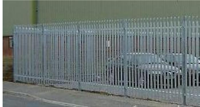
Figure 10: Typical galvanized palisade fence
