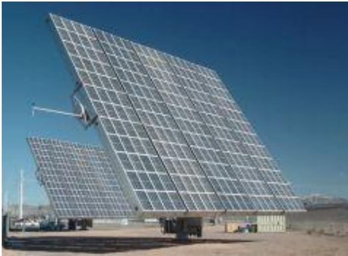
**Figure 4: Typical CPV Unit**
