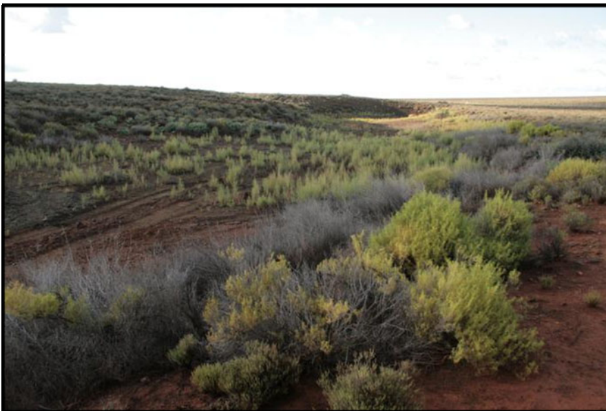
Figure 12. Borrow Pit 2 showing the existing excavation invaded by weedy pioneer species, notably Dittrichia graveolens and Galenia africana .
