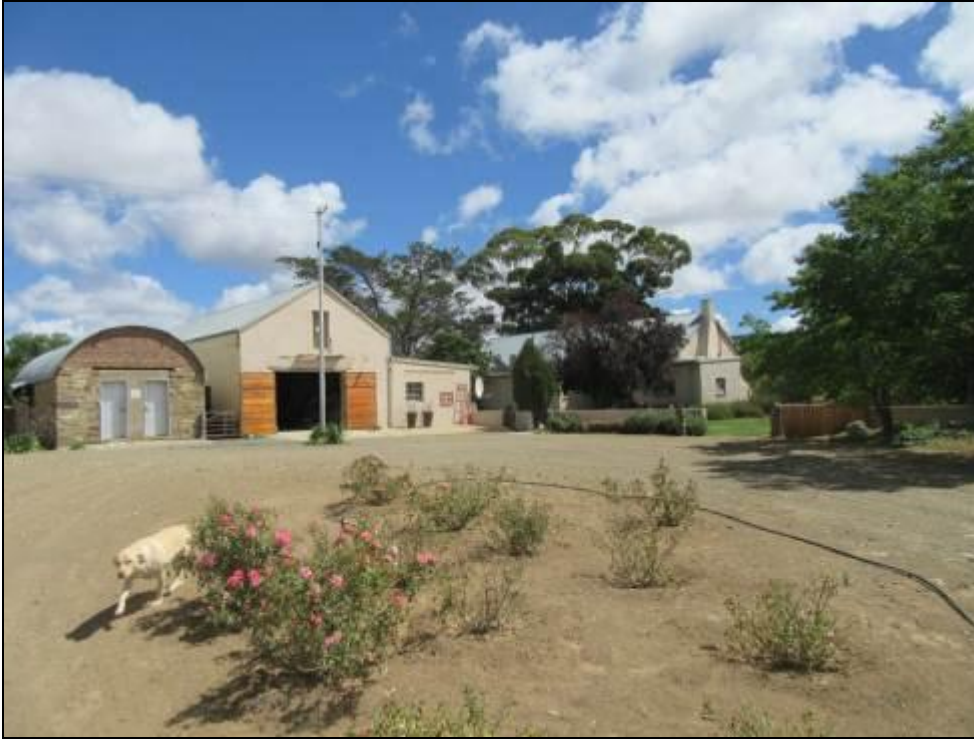
Photograph 1.6: Farm house and outbuildings on Fortuin farmstead
