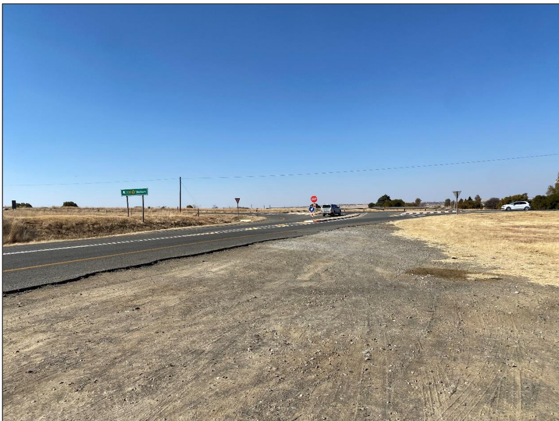
Figure 3.12: Power Line will cross over the R708.
