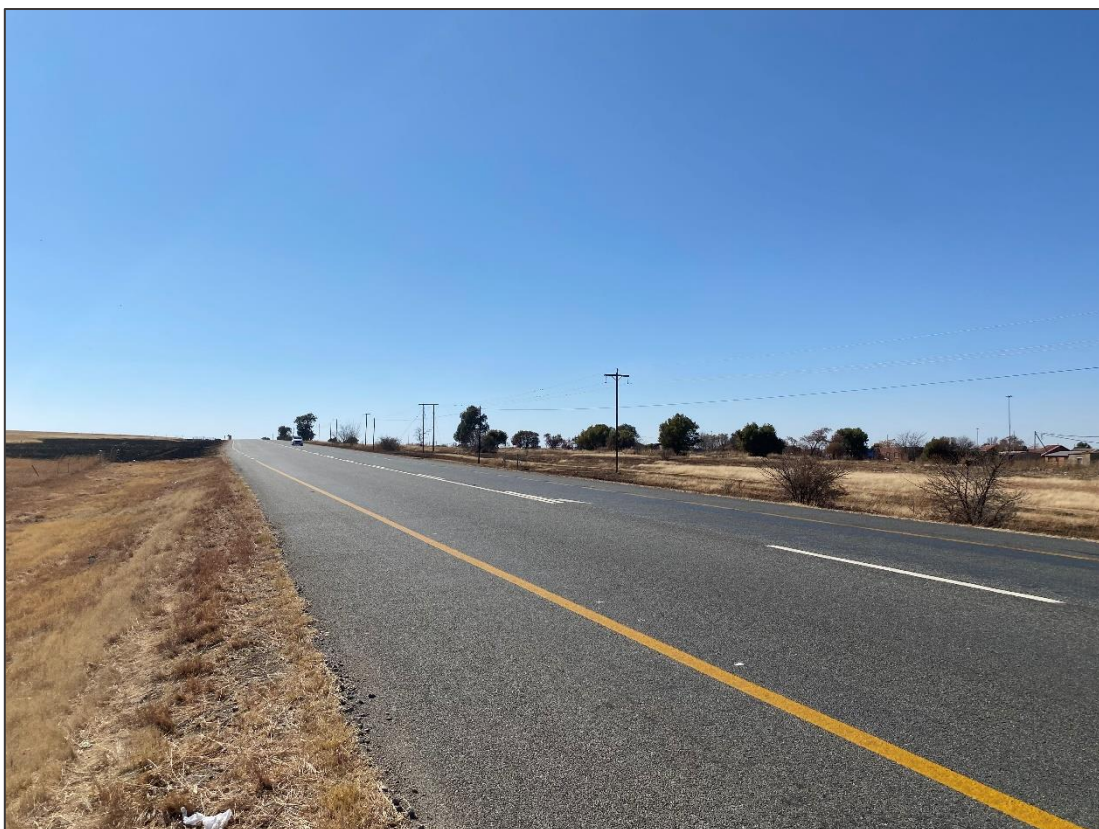
Figure 3.4: View of the R30 and a portion of power line corridor taken towards the north.
