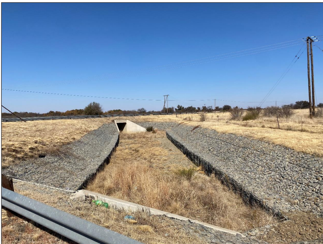
Figure 3.18: The proposed power line will cross over a storm water channel and the S478.
