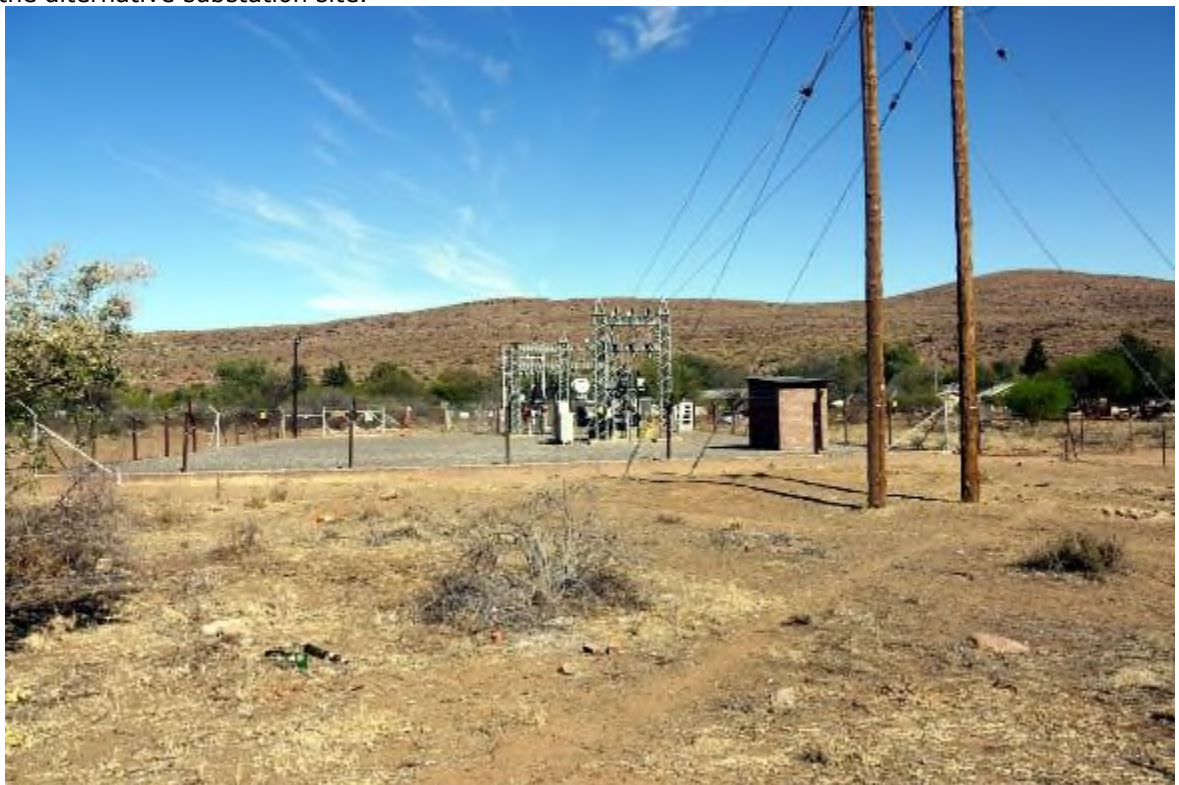
Plate 25 – VP10 looking west towards the existing substation.
