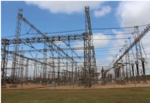
Plate 1 - Sub-station Bus Bars maximum height 10-15m
