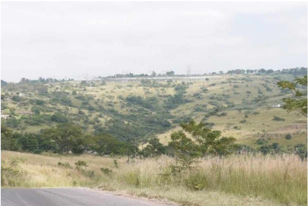
Plate 15, Distance view (1.5-2.0km) of the existing Hammersdale 400kV Sub Station. Note the 400kV pylons entering the site are the most obvious elements
