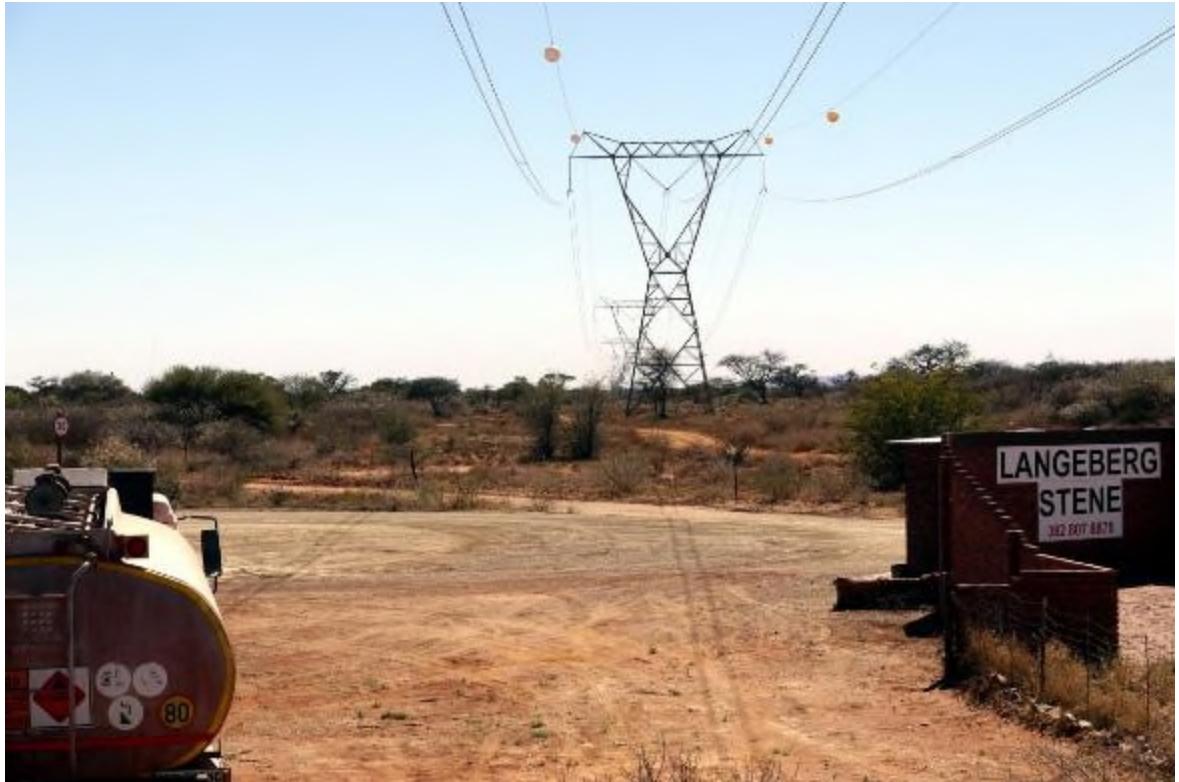
Plate 20 – VP5 located on the N14 at the crossing point of the existing 400kV overhead power line looking north east along the line.
