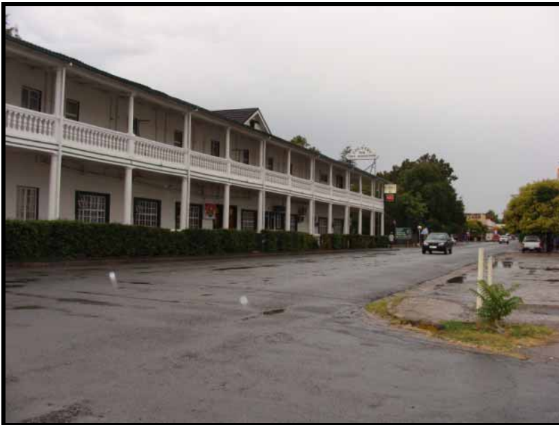
Photograph 2.1: View of Meintjies Street (N10), the main thoroughfare through Middelburg
