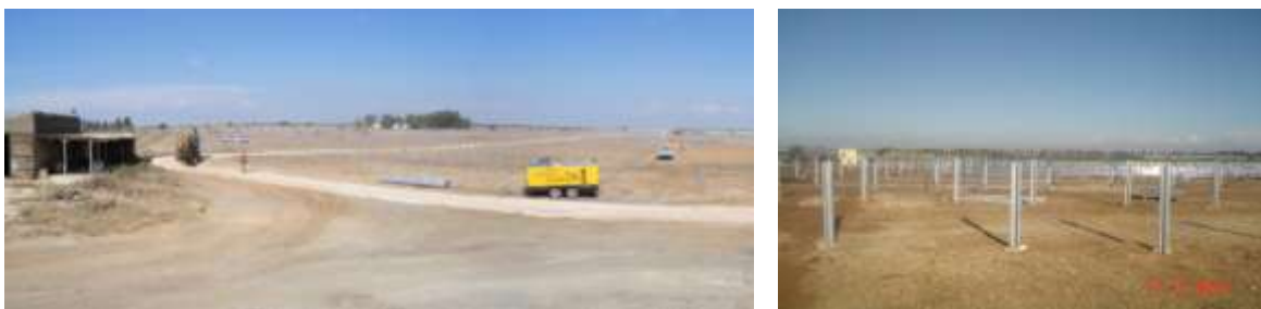
Figure 12: Illustration of a typical site after preparation
