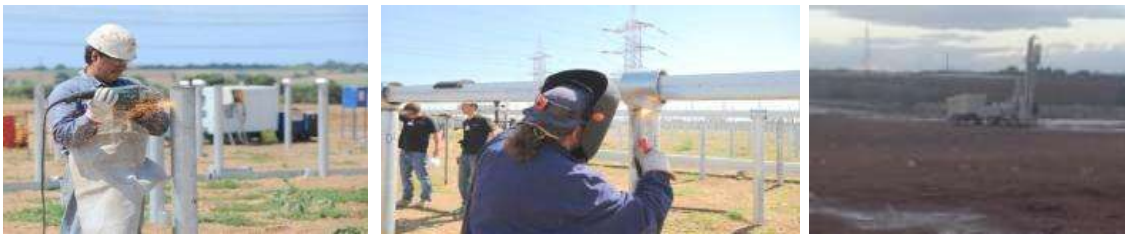
Figure 13: On-site construction of the PV arrays
