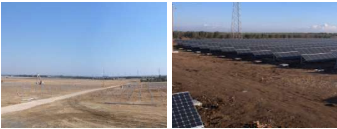
Figure 6: Typical internal road example
