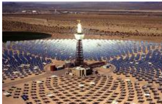
Figure 10: Example site of a CSP Solar Facility
