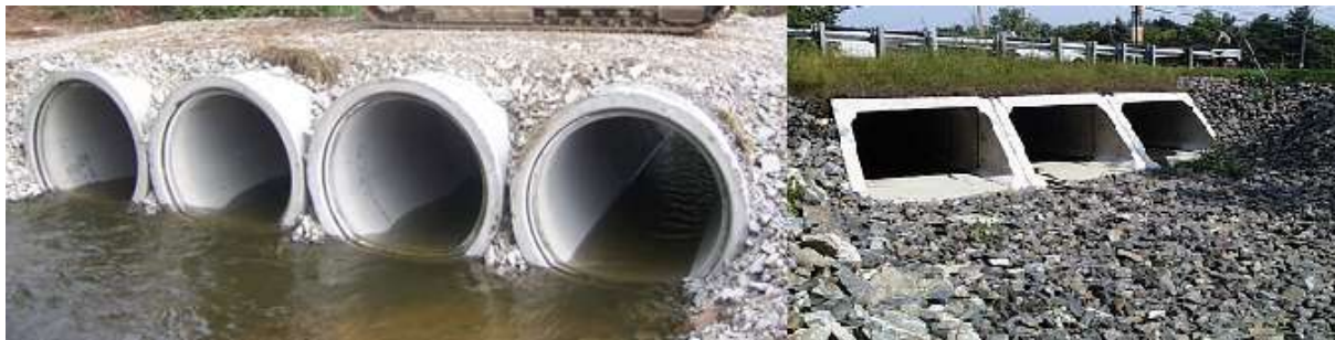
Figure 22 Installed concrete pipes and culverts
