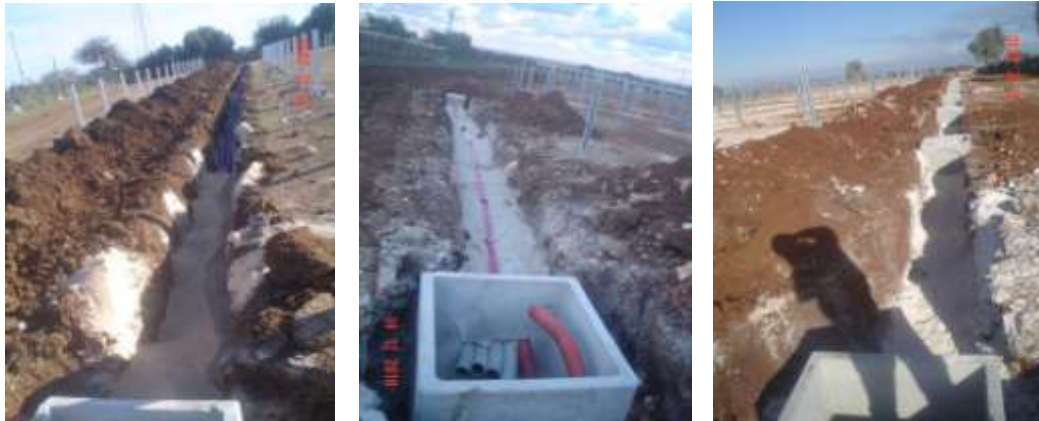
Figure 8: Typical cable trenches
