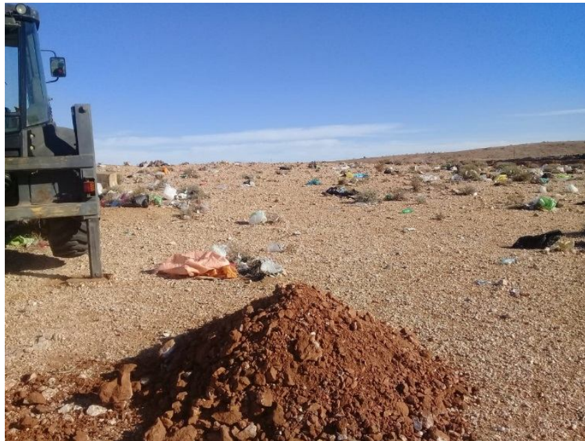
Trial hole 3 – Excavated material
