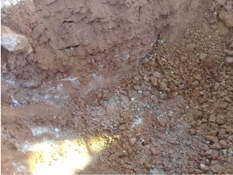
Trial hole 3 – 0,50 meter in depth
