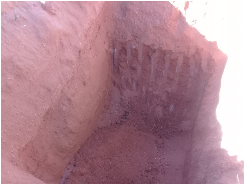
Trial hole 1 – 2,0 meter in depth
