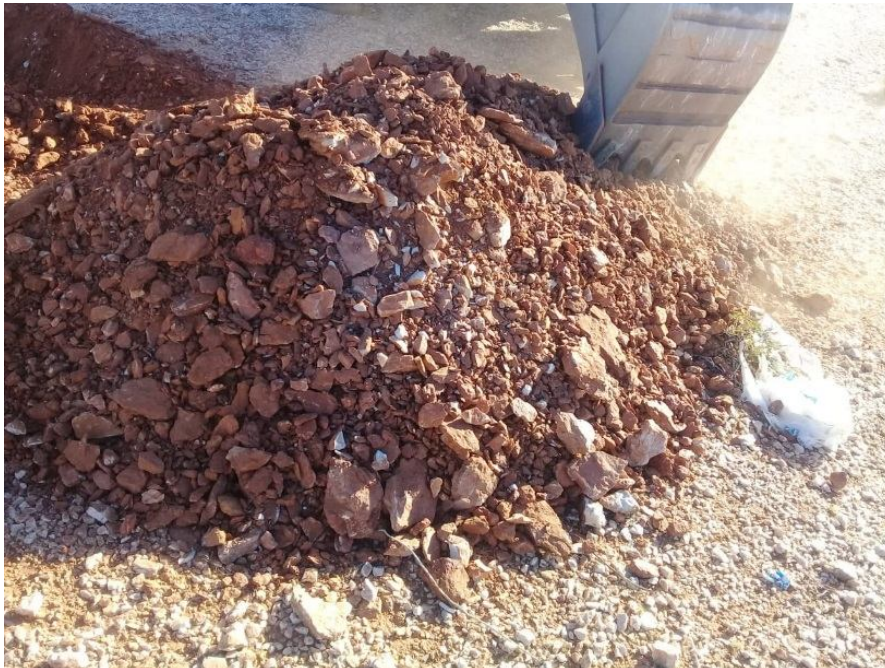
Trial hole 2 – Excavated material
