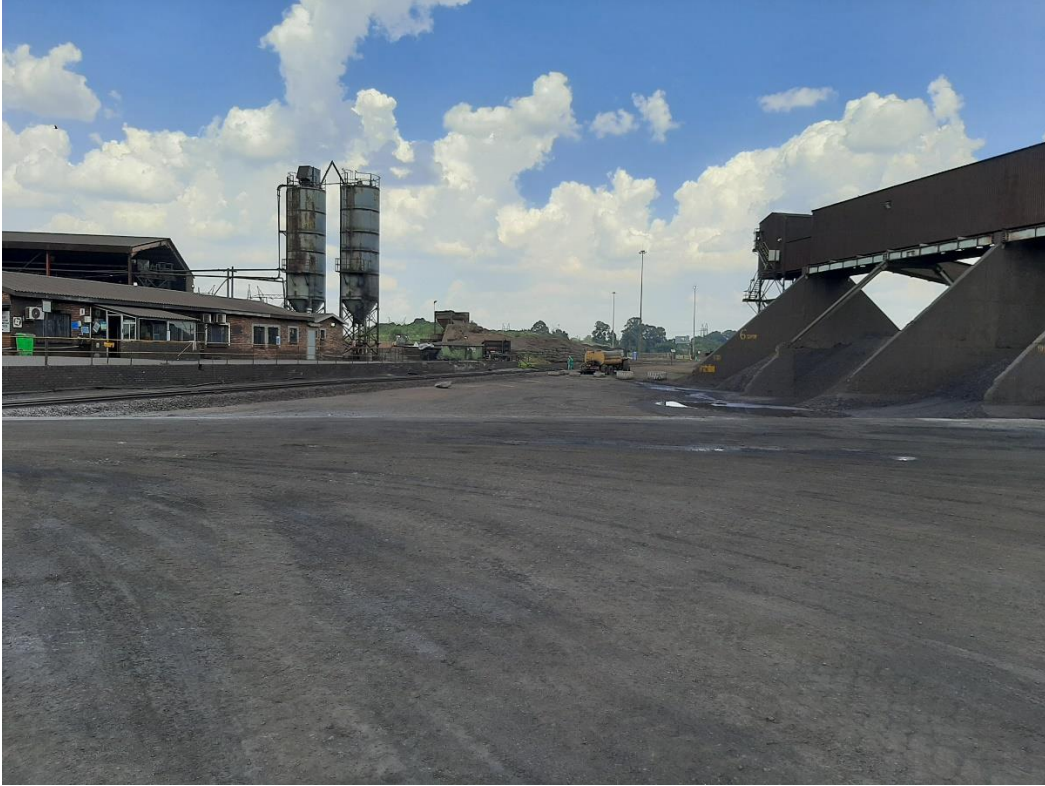
Figure 10: 25°53'50.5"S 29°07'02.3"E facing southeast
