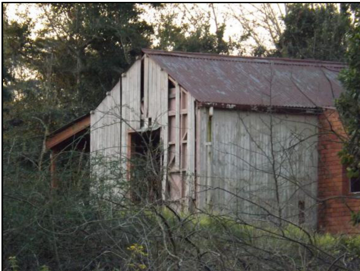
Plate 4. Corrugated house removed from York Village and transported to the then Midmar Historical Village at Howick. Poor management practices is evident and the loss of a heritage.
