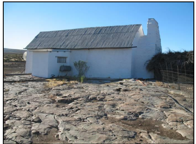
Figure 18. Node 6 Hunting lodge (back). Note bathroom addition
